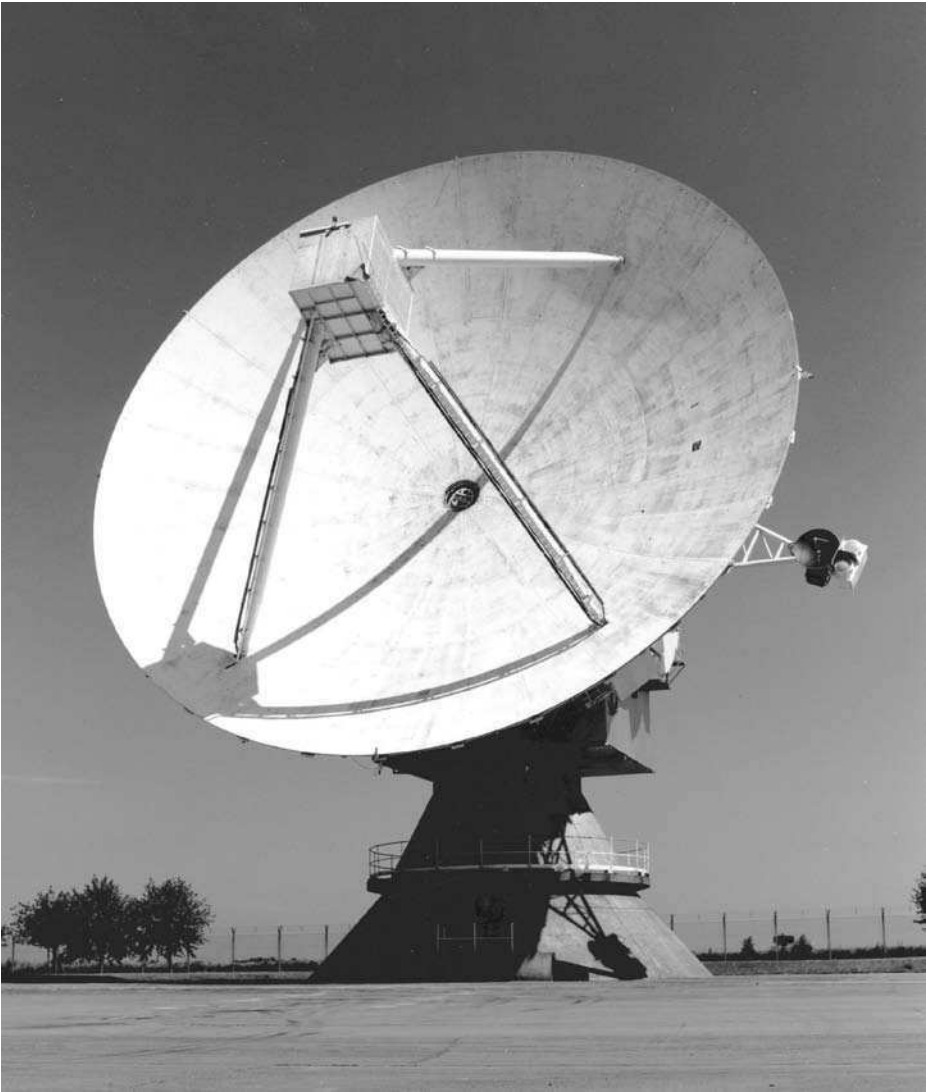
Figure 10.3 This 25-metre, 3 GHz radar at Chilbolton in the UK is used for research into the effects of weather, in particular precipitation, on radio communication, both terrestrial and satellite. It is the largest steerable meteorological radar in the world, measuring raindrops and clear-air turbulence. To the right are two much smaller antennas operating at 35 and 94 GHz for the measurement of cloud droplets. Photograph courtesy of the Council for the Central Laboratory of the Research Councils (CCLRC).
