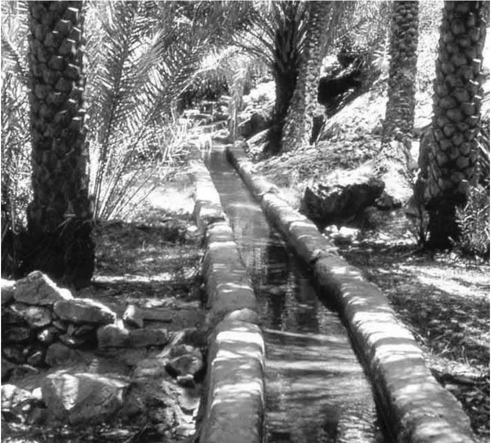
Figure 1.1 This ‘falage’ flows though a remote village in northern Oman, fed from a spring in the mountainside. It fulfils all the needs of the villagers from domestic water supply to irrigation of the palms. Such falages have been in use for millennia in the arid regions of the Middle East.
